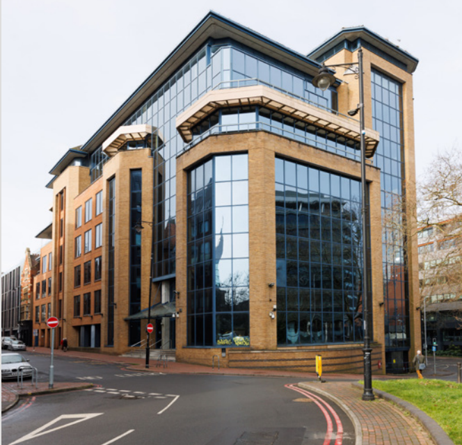
NORTH GATE HOUSE
